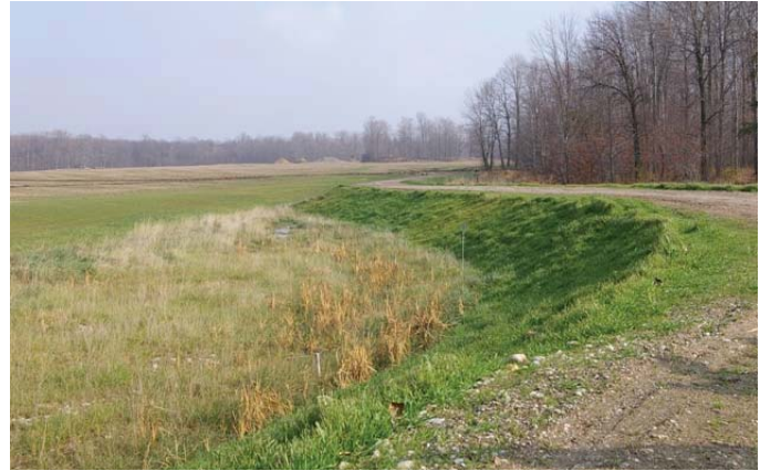
Sediment Control Berm
