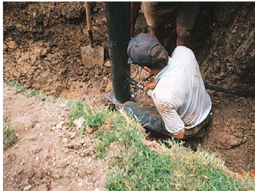
Consult a licensed water well contractor for advice and assistance with the extension of the water well casing.
