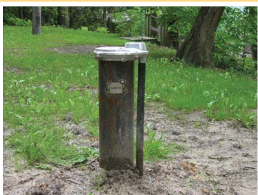
Regrade soil around the well to prevent surface water from ponding near the casing.
