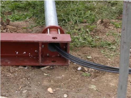
As you can see the tower base is constructed with a hinge design to facilitate raising and lowering. A gin pole which is half the height of the tower is inserted into the base at a right angle to the tower. The cables from the front anchor are transferred over to this pole which acts as a lever. A cable is then attached to the
