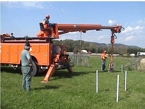
The tower sits on a concrete base with 4 guy wire assemblies connected to 4 outlying pillars. The tops of each of these must be at the same level. Milton Hydro generously donated the use of one of their auger trucks to drill the holes in which we used 24" Sono Tubes as forms. The two pillars to the left and right of the centre are slightly ahead of the centre line of the base so that the cables attached to them loosen as soon as you start to drop the tower.
