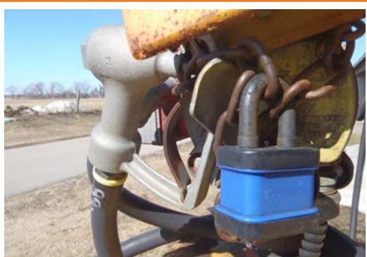
A locked fuel storage will help to prevent unauthorized access.
