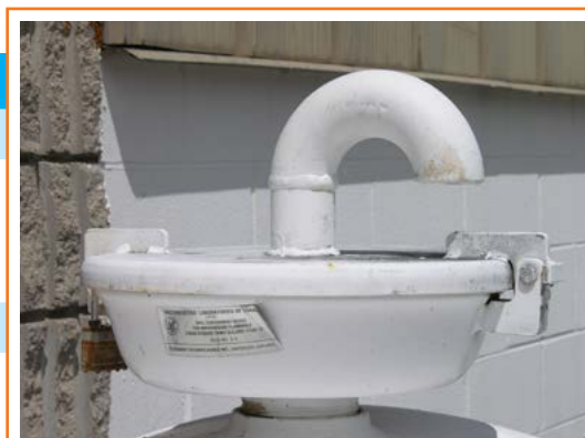
The overfill device is designed to prevent filling to more than 95% capacity.
