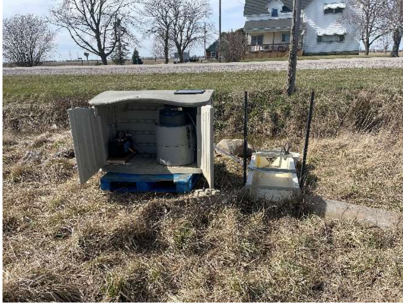
Figure 5. Merlin A's flume (right) capturing surface flow entering the municipal drain, with the permanent ISCO enclosure to the left.
