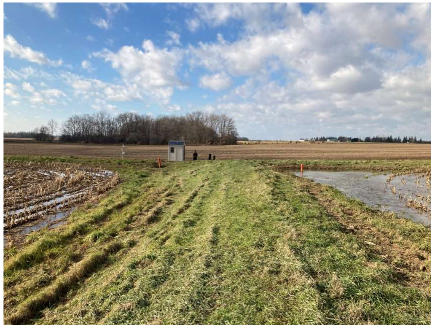
Figure 11. Photo of T-shaped berm separating the two monitored catchments at the North Kettle EOF.
