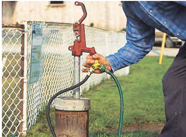
This drilled well metal casing has a frost-free hydrant faucet with an anti-backflow device.
