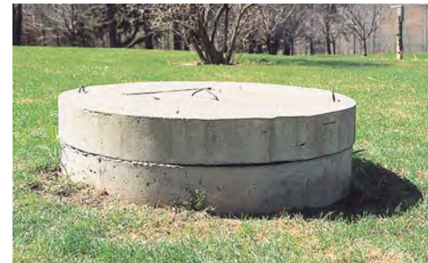
Bored/dug wells with concrete lids are considered vented.
