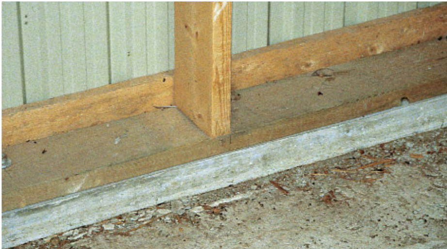
An impermeable floor with curb will contain spills for ease of cleanup.
