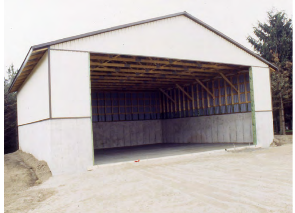
A permanent roof is the best way to keep rainwater out of the mixing/loading area.
