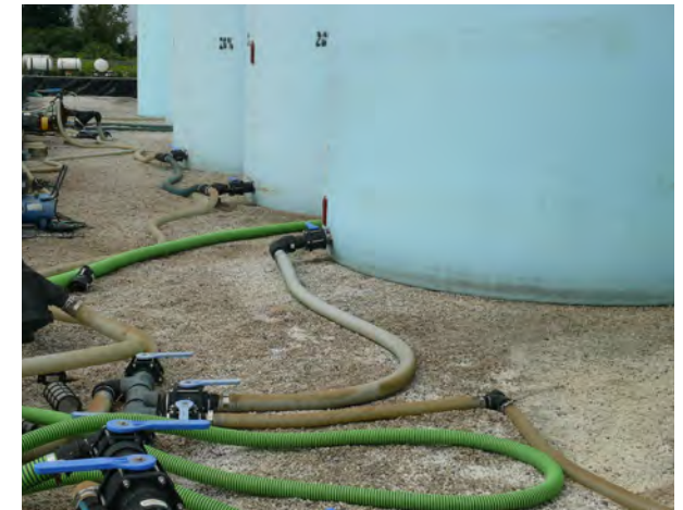
A closed system for product transfer reduces the risk of a spill.
