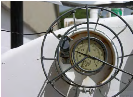
A vacuum reading indicates that both walls of a double-walled tank are sealed.
