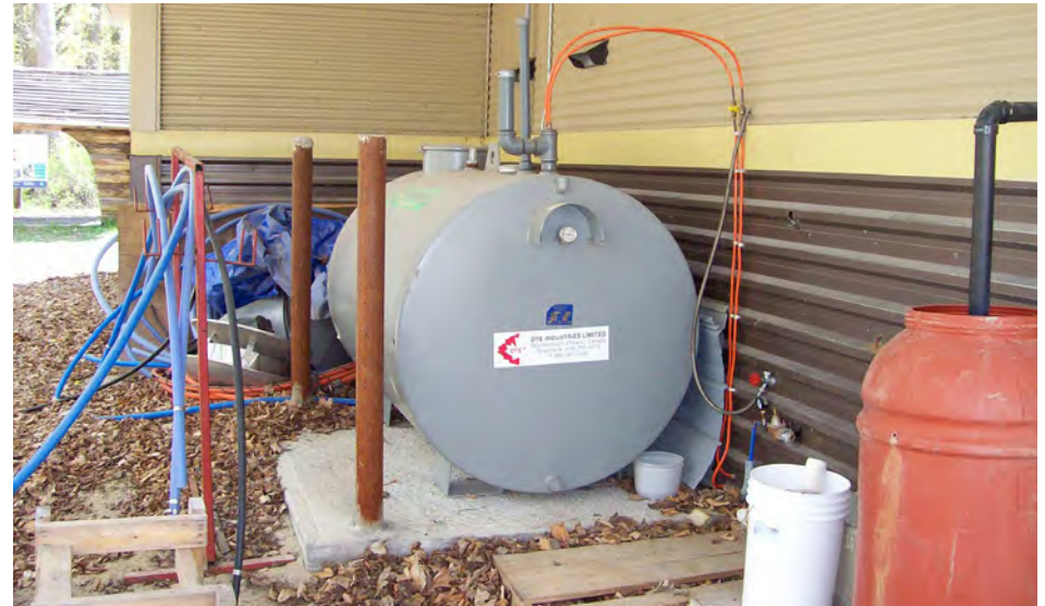
Fuel delivery lines are often the source of leaks.
