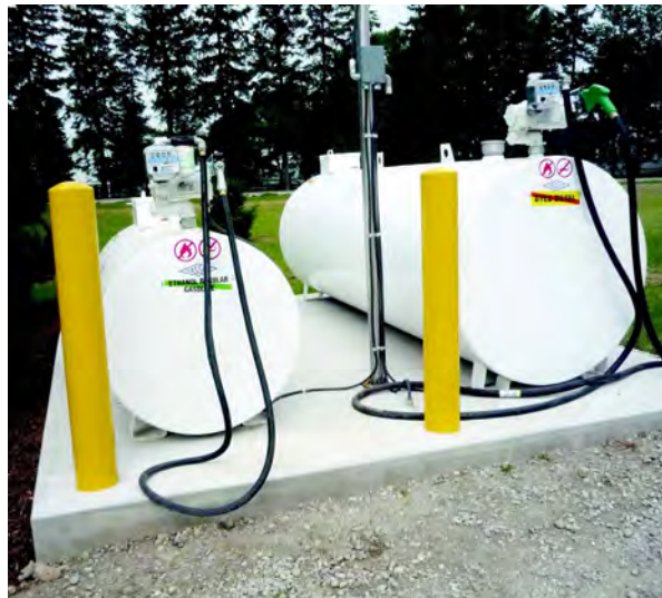
Bollards in place along travel lane to protect fuel storage tanks from vehicle impact.
