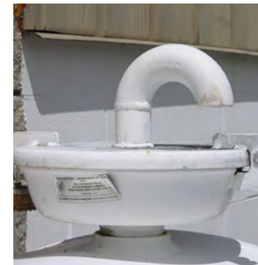
The overfill device is designed to prevent filling to more than 95% capacity.
