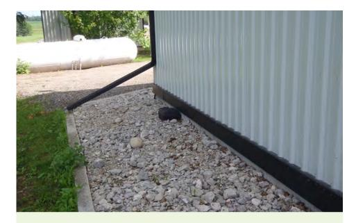
Eavestroughs, foundation and footing drains should not be connected to the sewage system.
