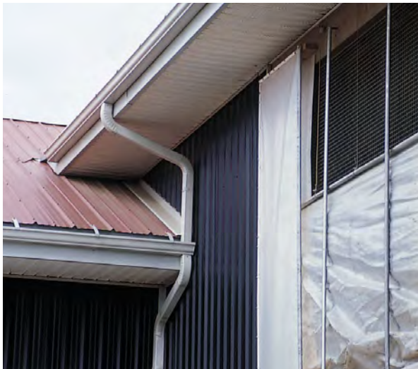
A properly designed eavestrough system will direct clean water away from storage or yard areas.
