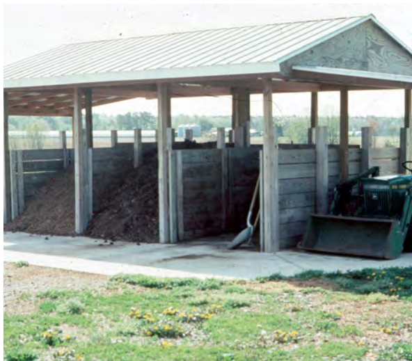
A roofed compost site will divert clean water from mixing with compost and producing runoff.
