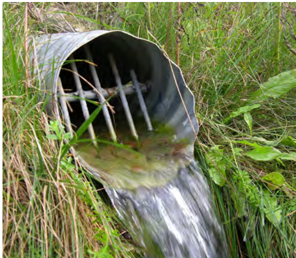
Drainage tiles are a conduit to surface water, and composting sites should be located at least 10 m (33 ft.) away.
