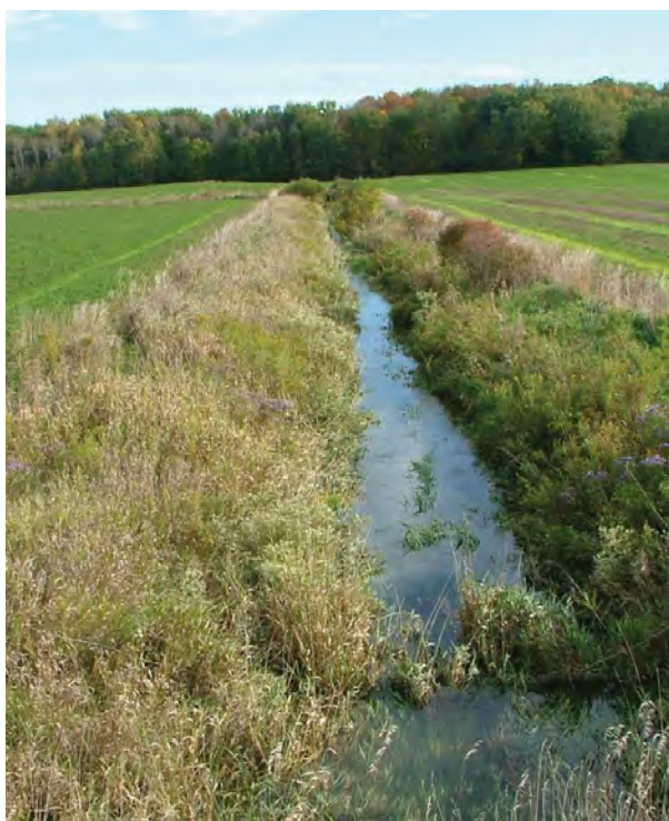
A thick cover of vegetation will stabilize the banks and greatly reduce maintenance requirements.
