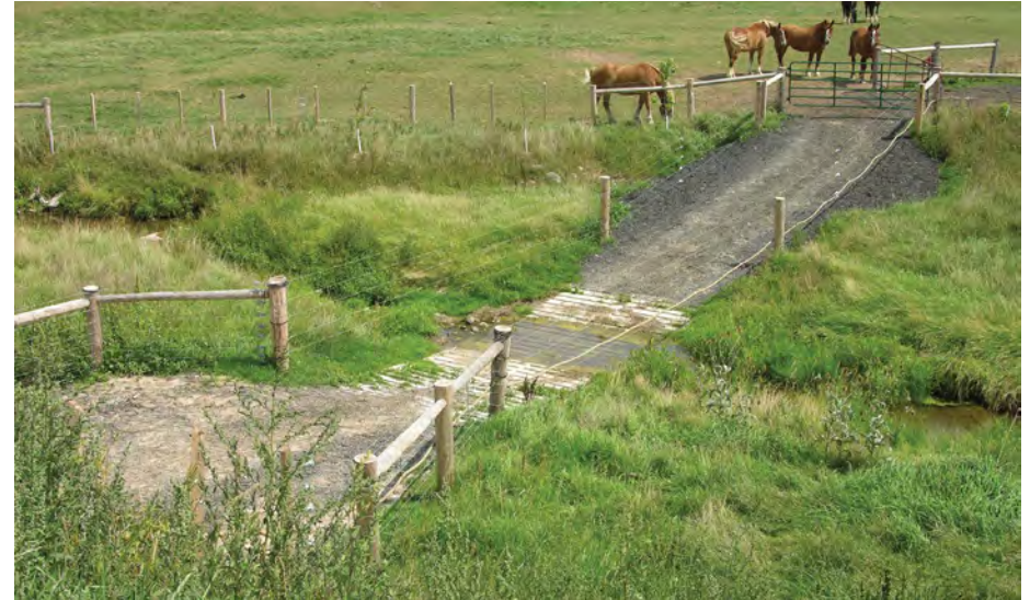
A fenced, bed-level crossing will manage livestock impact on the watercourse while providing access to pastures.
