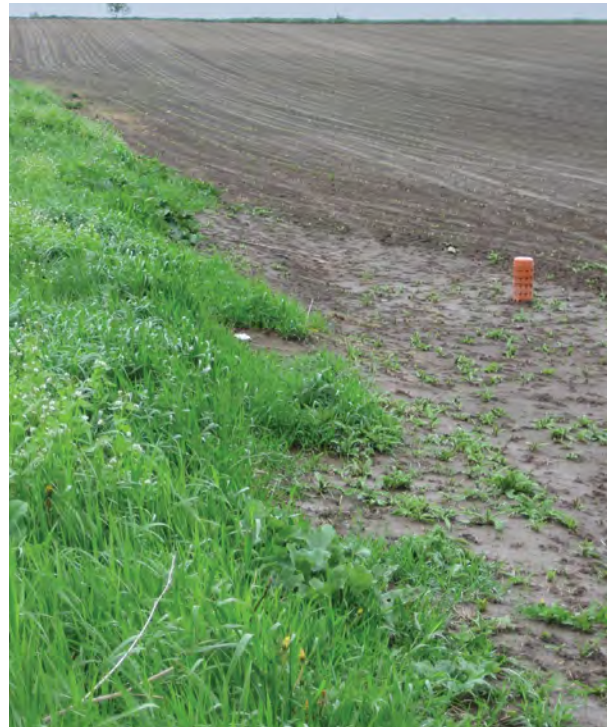
Surface inlets move excess surface water on cropland to subsurface drainage systems in a controlled manner that reduces soil loss.
