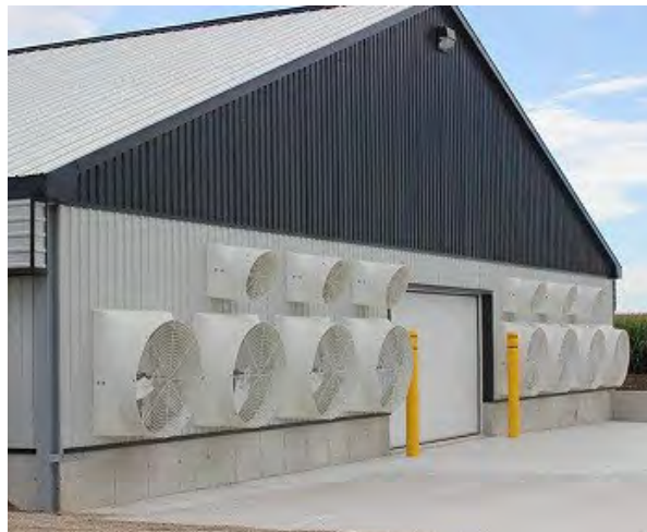
Tunnel exhaust fan bank in broiler barn.
