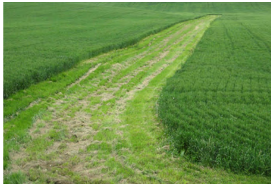
Landscape and constructed features, such as grassed waterways, are an important part of a strategy to manage extreme overland flows of water.
